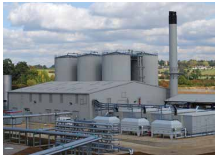
..... Steam application for water treatment facility.
